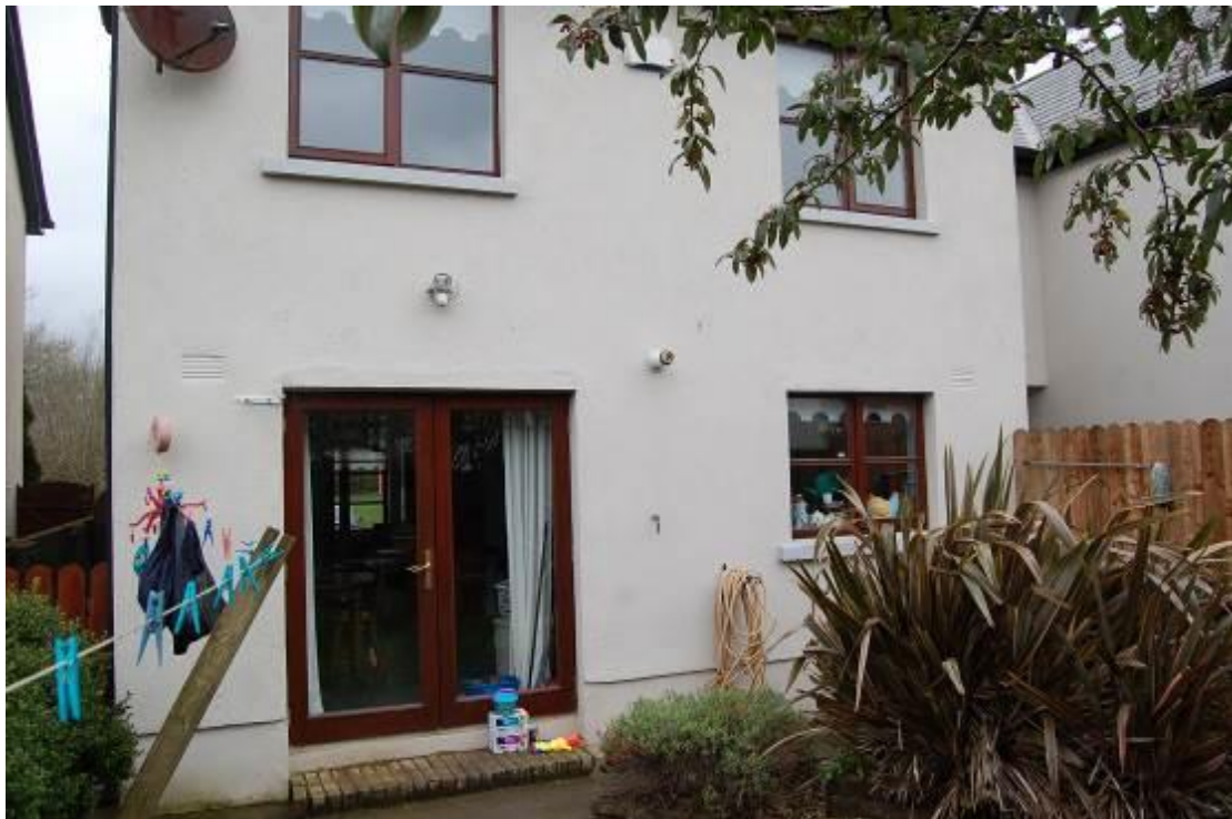
Photo 1 General View Rear Elevation
