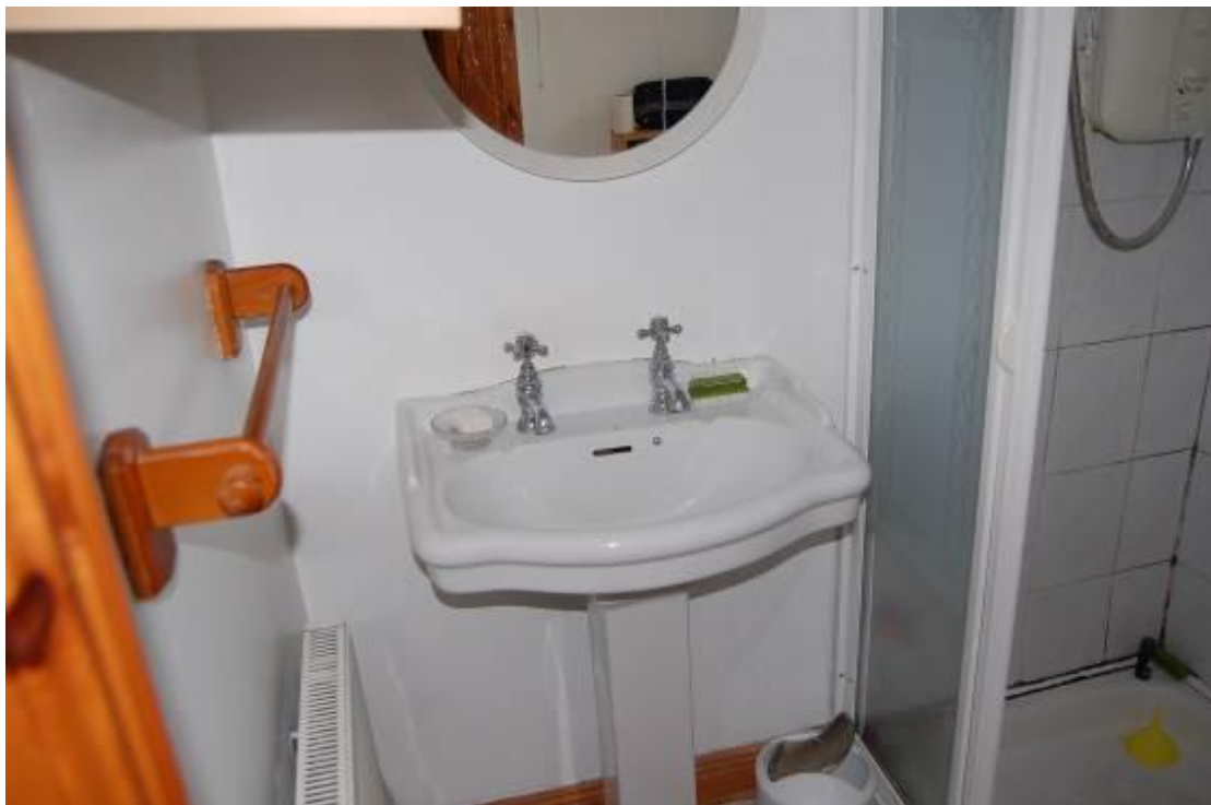
Photo 8 Tap to WHB to be Repaired
