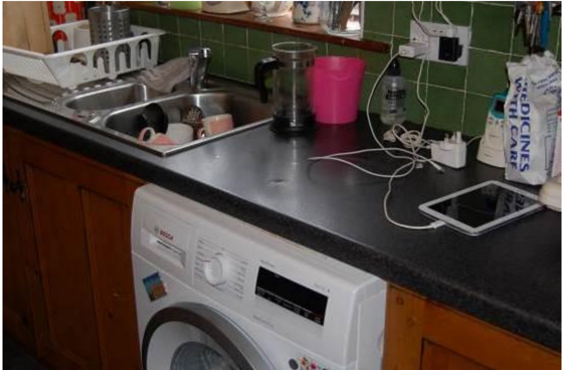
Photo 9 Some damage to Kitchen Worktop
