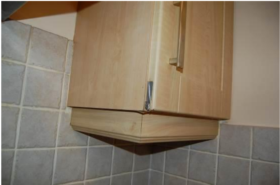
Photo 4 Damage to Corners of Doors (typical)
